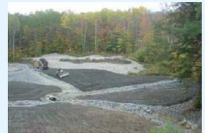
Designs for backfilling, grading and stabilizing a 3-acre basin affected by mining waste at the Elizabeth Mine NPL site in South Strafford, Vermont, included intent to mirror the site's natural contours and drainage patterns. The fully graded surfaces were seeded with native plant species that target Vermont state conservation and wildlife goals.
