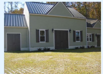
Design and construction of an offsite groundwater treatment plant near the Lawrence Aviation Industries site in Port Jefferson Station, New York, included installation of:
