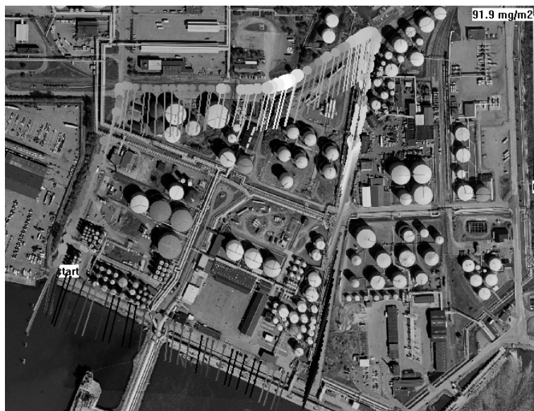
Figure 63. SOF measurement on 17-May-2004, 30 minutes after having completed pumping of gasoline containing drainage water to a tank. (Aerial photo: Copyright Lantmäteriet 2004-11-09. Ur Din Karta och SverigeBilden)
