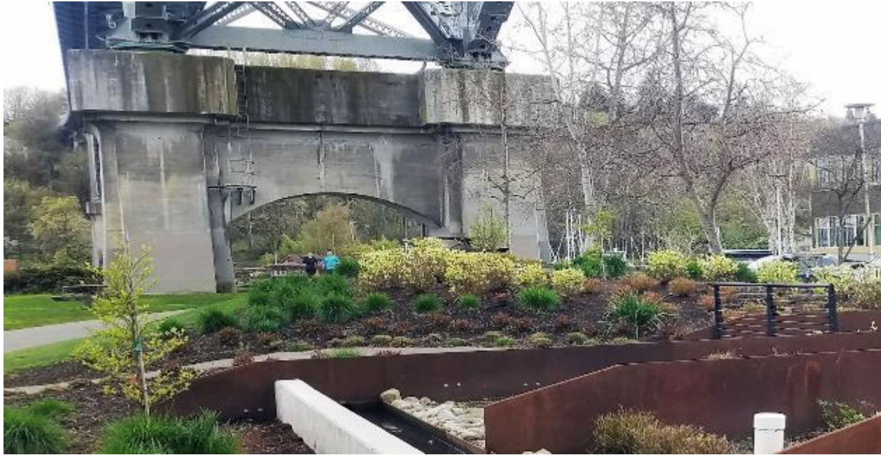
Green stormwater infrastructure capturing and treating runoff from heavily-trafficked highway bridge in Seattle.
