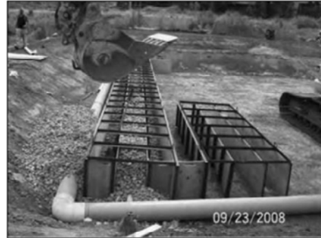
Construction of the BCR in Park City, UT Photo courtesy Jeff Schoenbacher Park City Municipal Corporation
