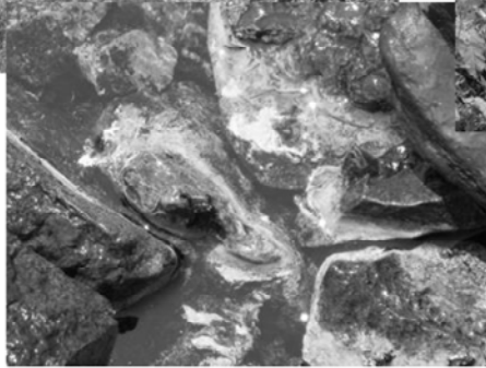
Outfall from Penn Hills BCR
