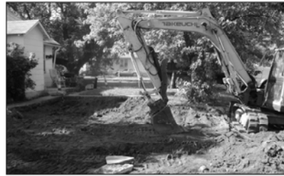
Post-Excavation Confirmatory Sampling
