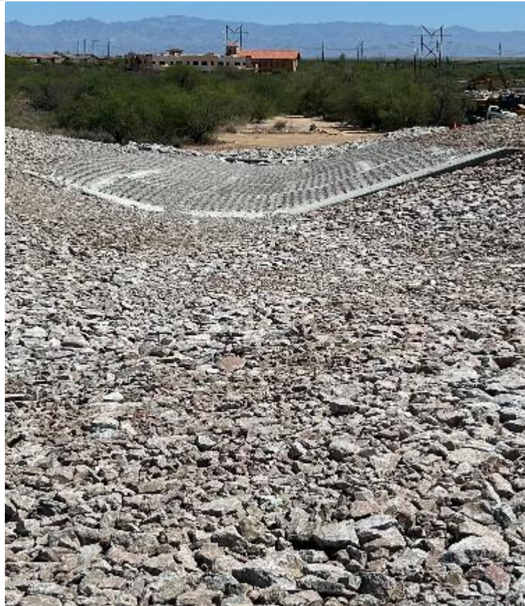
Articulated Concrete Block at Eagle Picher Mill. MW-1, Figure 6-1
