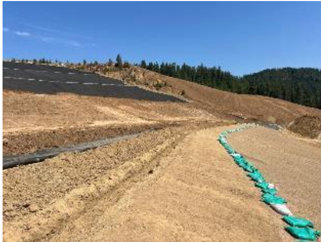
Geomembrane Bedding at Midnite Mine Superfund Site, WA
