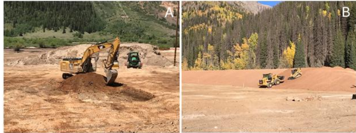
MIW Treatment Sludge Blending with Tailings at Bonita Peak Superfund Site, CO
