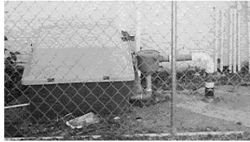
Figure 6-1. Small-scale soil vapor extraction (SVE) system designed to address the source of vapors. Photo Source: Vapor Mitigation Sciences, LLC.
