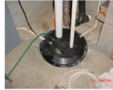
Figure J-4. Passive sump mitigation system. Photo Source: Kansas Dept. of Health and Environment
