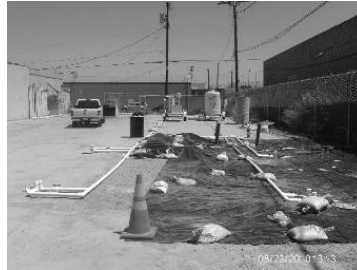
Sump removal at a plating shop
