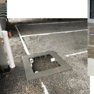
Passive Sub-Slab Venting (SSV) Systems Epoxy Floor Coatings (EFCs)
