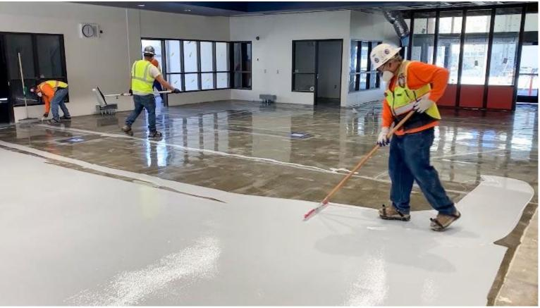
Figure 1 of Epoxy Floor Coatings Technology Information Sheet.
