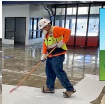
Epoxy Floor Coatings (EFCs)
