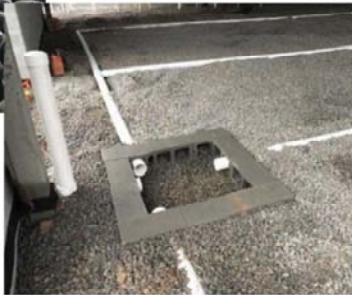
Passive Sub-Slab Venting (SSV) Systems
