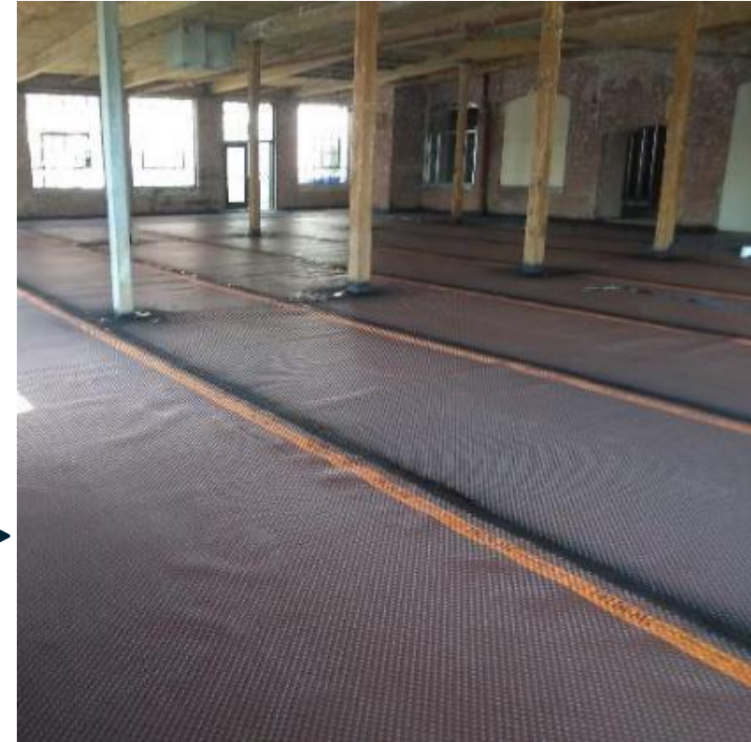
Source: Contractors Waterproofing, 2021. Used with permission.
