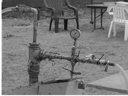
Temperature and Pressure Gauges
