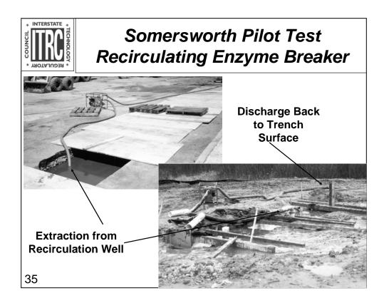
Enzyme breaker is added to trench surface, into extraction wells, and/or through injection points or other wells.
