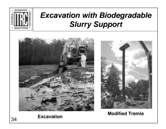
Biodegradable slurry level is maintained above groundwater table to provide hydraulic head on trench.
