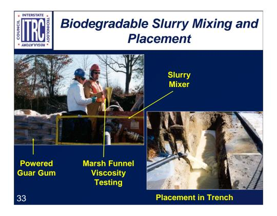
Guar gum in powered form is mixed with water in a slurry mixer.
