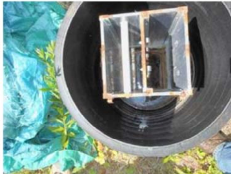
Adjustable Elevation Head Weir for BCR Effluent
