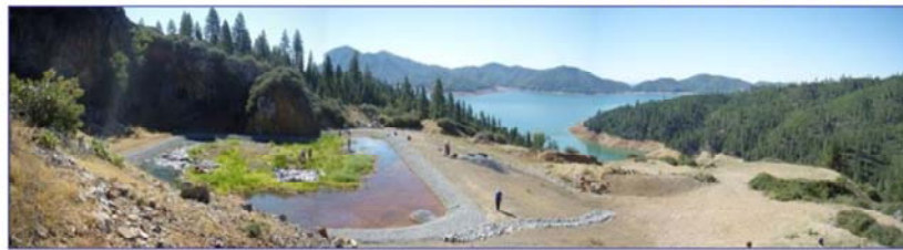
Golinsky Mine, Shasta County, CA Biochemical Reactor Photo Courtesy of Douglas Bacon
