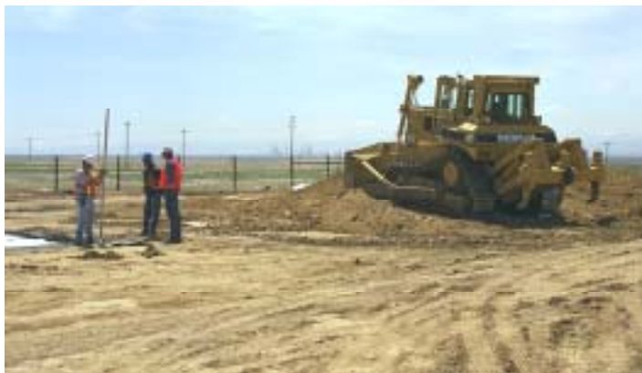
Figure 5-1. Placing soil lift for test pad construction at the Rocky Mountain Arsenal.
