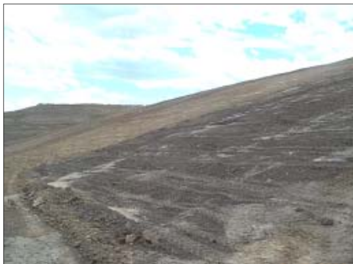
Figure 5-6. Intermediate cover (dark soil) at Denver Arapahoe Disposal Site, alternative cover layer placement (light soil) in the distance.
