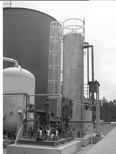
Fluidized Bed Reactors at Longhorn Army Ammunition Plant
