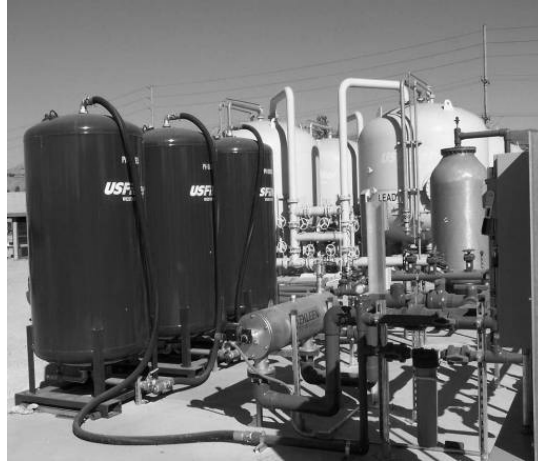
Three vessels at Fontana, CA site
