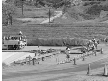
Former Munitions Facility California
