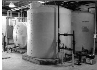
Dual-Phase Continuous-Flow Stirred-Tank Reactor (CSTR) system at Pyrodex Plant, Herington, KS
