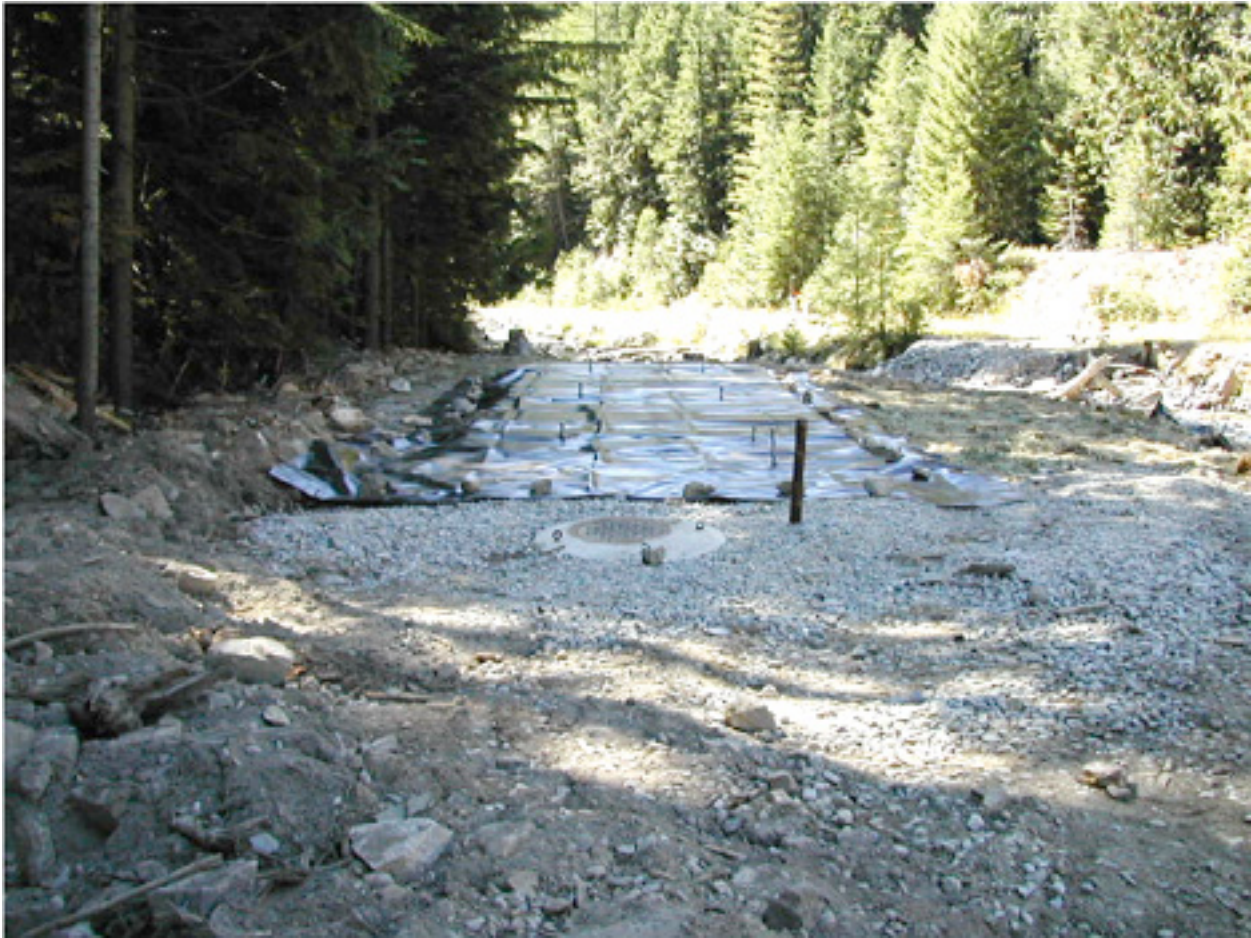
Figure 10. Final emplaced Apatite II PRB at Success Mine between East Fork of Ninemile Creek and the Tailings Pile in September 2002.
