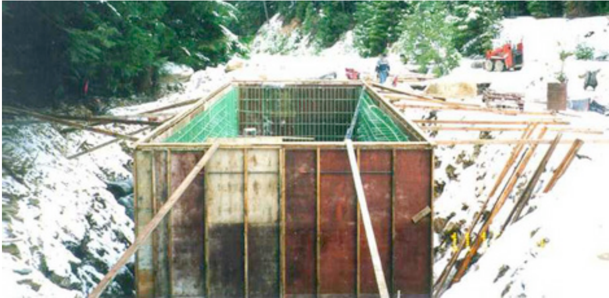
Figure 9. Construction of PRB vault between East Fork of Ninemile Creek and the Tailings Pile in January 2000.
