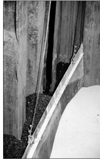
Gravel and Zeolite Placement
