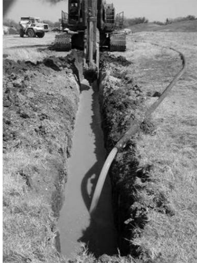
Biopolymer slurry wall installation
