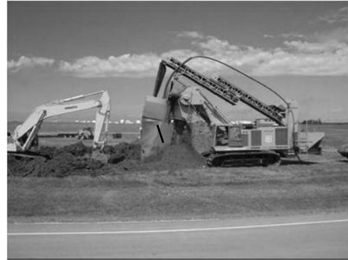
One-Pass Biowall Installation at Ellsworth AFB, South Dakota
