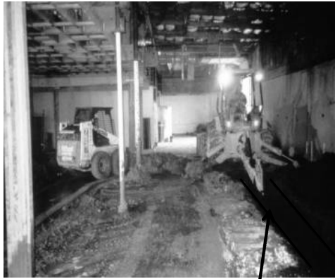
PRB Trench Within Building
