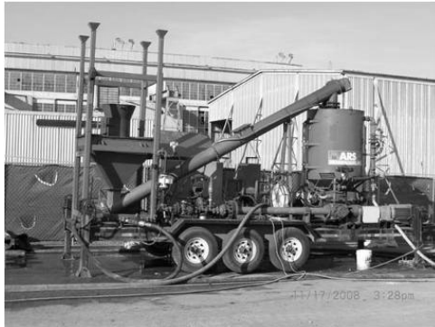
ZVI injection at Hunters Point Shipyard Parcel G, November 2008
