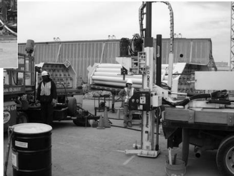
ZVI injection at Hunters Point Shipyard Parcel G, November 2008
