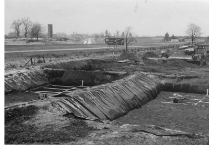
PRB-5: Figure 6-1. Horizontal PRB - treatment of septic system nitrate (Courtesy of Septech, Inc., 2003)
