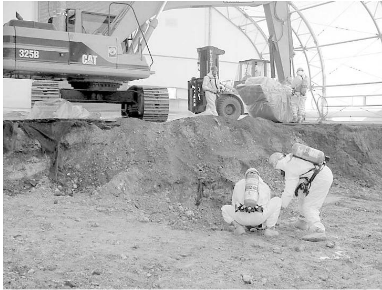
Removal of plutonium-contaminated soil occurred under large, moveable tent structures.
