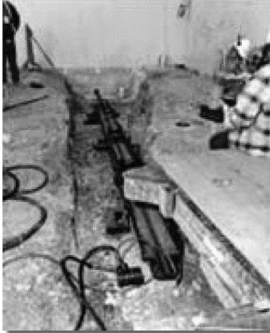
Environmental sampling using HDD at Building 865 at Rocky Flats.
