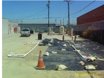
Sump removal at a plating shop
