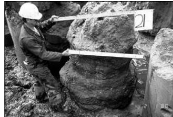
Excavation of S/S column
