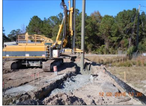
Installing Vertical Wall With A Panel Cutter
