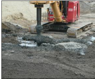
Auger mixing at a former MGP site.
