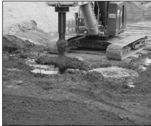
Auger mixing at a former MGP site.
