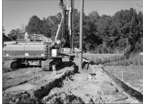
Installing Vertical Wall With A Panel Cutter
