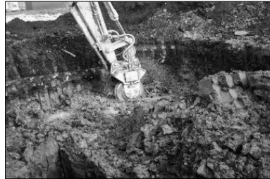
Treatment by rotary blender at former wood-preserving site Port Newark, NJ
