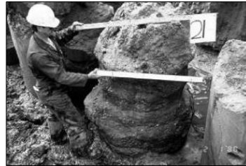
Excavation of S/S column
