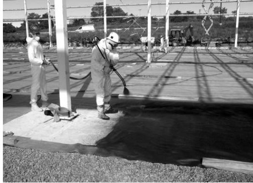
Spray on barrier being applied during construction. Photograph courtesy of LBI Technologies, Inc.
