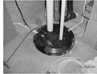
Passive sump mitigation system
