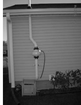
Active sub-slab depressurization (SSD) system
