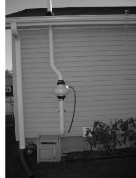
Active sub-slab depressurization (SSD) system
