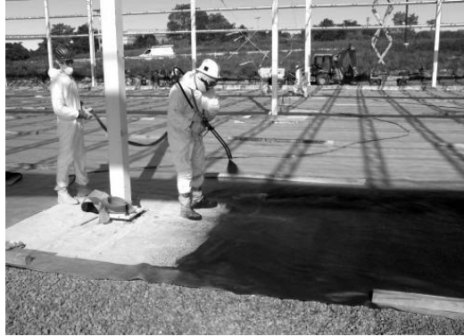
Spray on barrier being applied during construction. Photograph courtesy of LBI Technologies, Inc.
