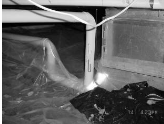
Crawlspace mitigation using sub-membrane depressurization (SMD)
