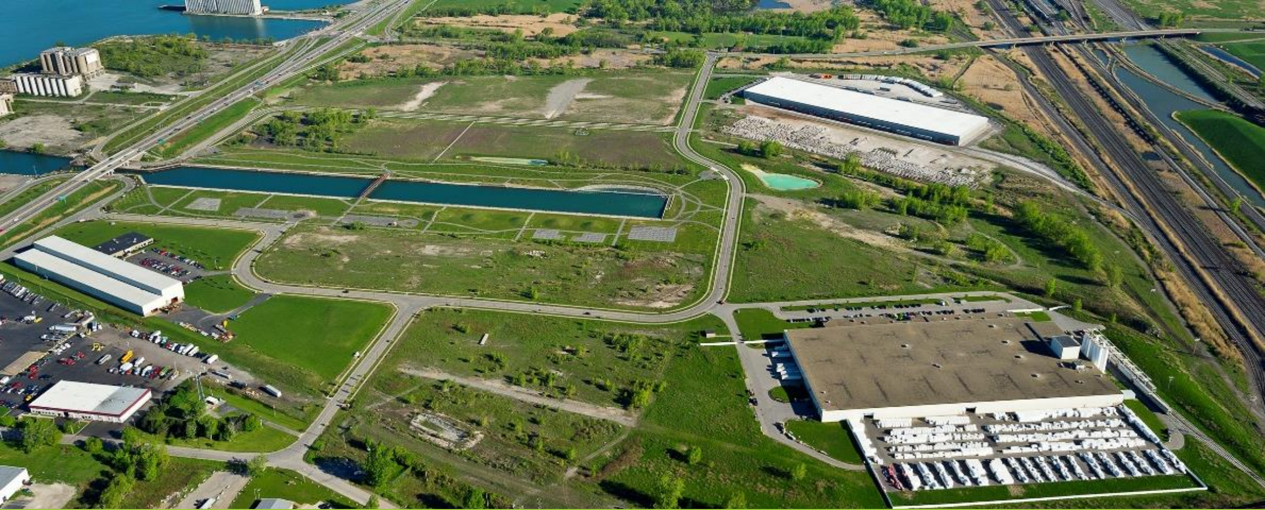
BUFFALO LAKESIDE COMMERCE PARK Former Hanna Furnace Pig Iron manufacturing facility
