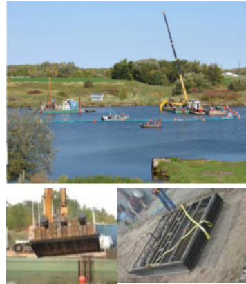
SLURRY INJECTION AND COVERED ROTOTILLER
