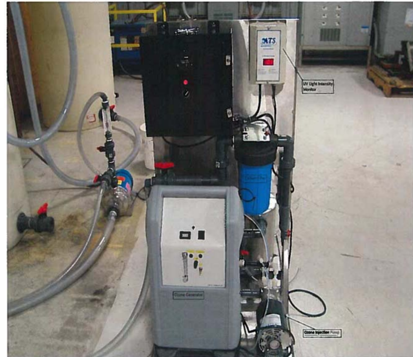
Figure 1.0 Front view of system showing the ozone generator, carbon post-filter and system controls:
