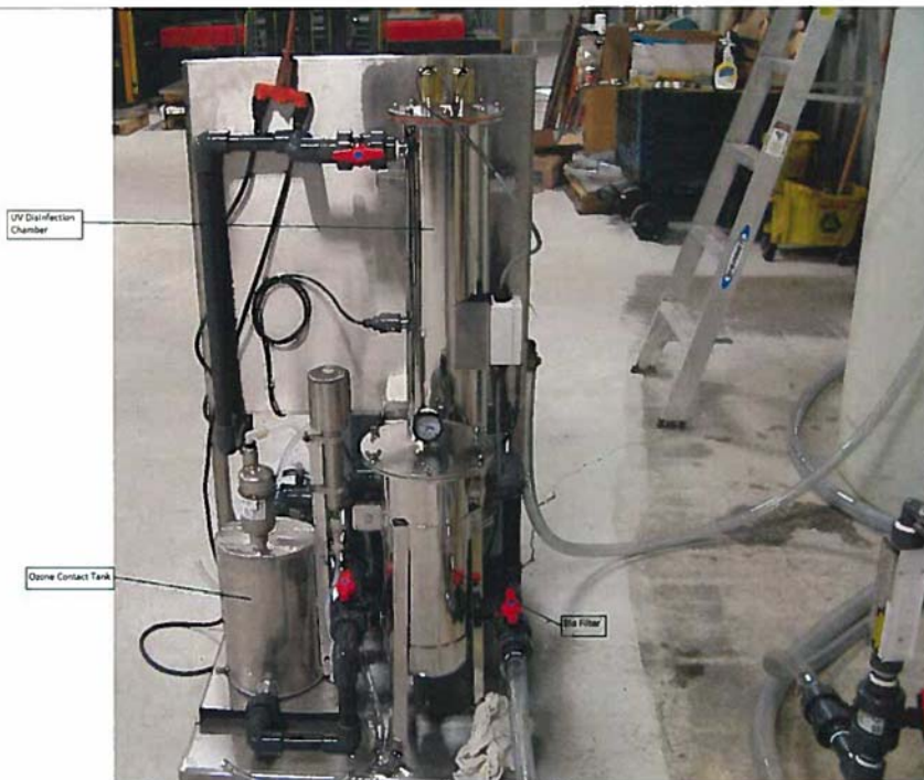
Figure 1.1 Rear view of system showing pre-filter, ozone contact tank and UV lamp chamber:
