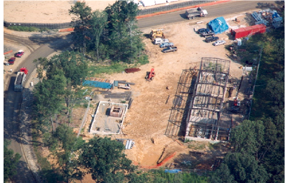
Aerial view of treatment plant under construction – August 25, 1994 NJDEP Closeout Report 6/2011
