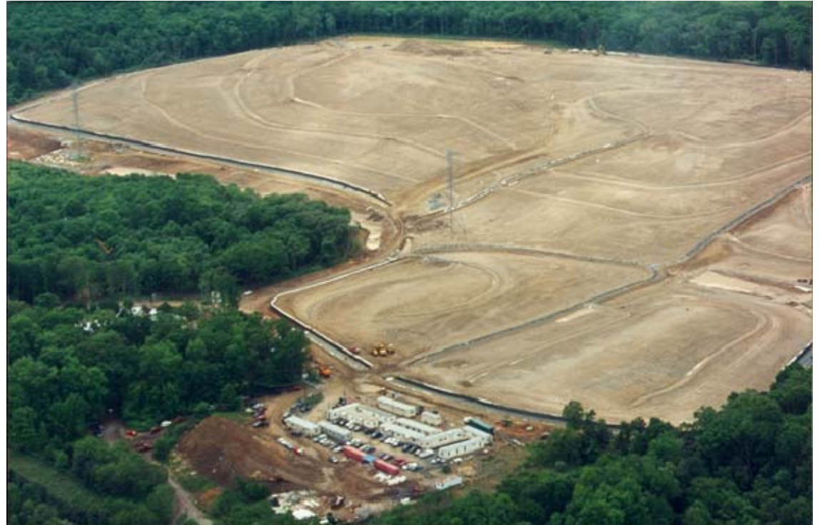
Aerial view of landfill looking west during construction – May 30, 1995 NJDEP Closeout Report 6/2011
