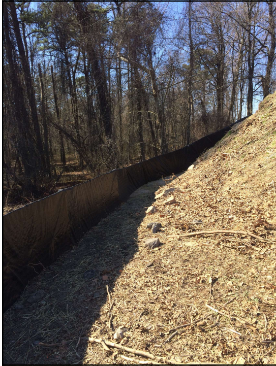
Protecting trees and installed super silt fence
