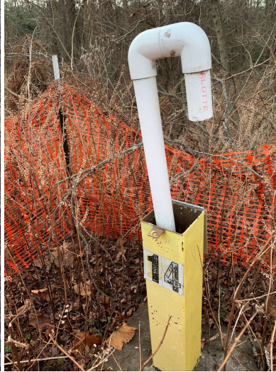
Typical Methane Monitoring Point
