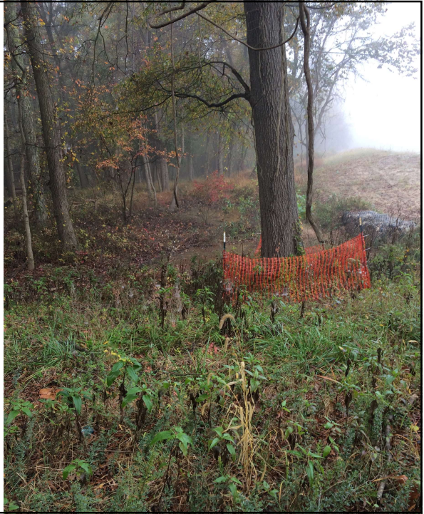
Protecting trees and installed super silt fence
