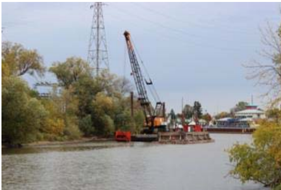
Crane operated environmental dredge bucket
