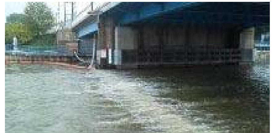
Silt bubble curtain installed at downstream extent of project (8 th Street Bridge).
