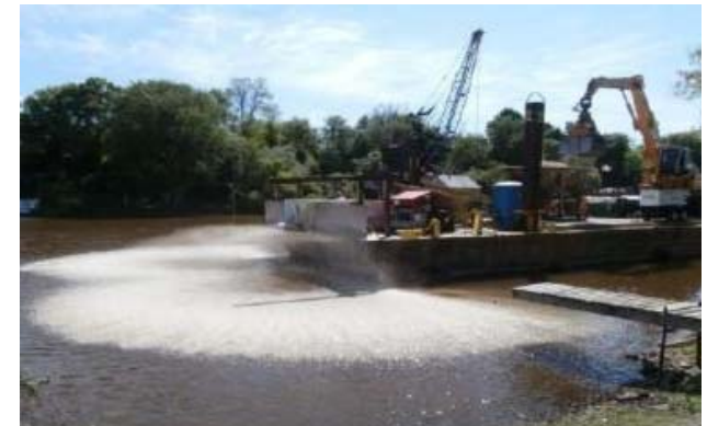
Post dredge residual management sand placement
