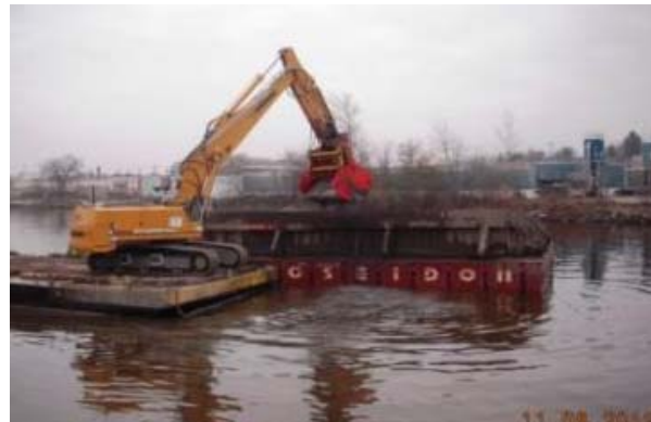
Excavator operated environmental dredge bucket
