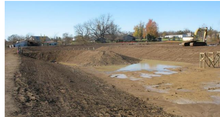
MRPTS oxidation cell under construction, fall 2008
