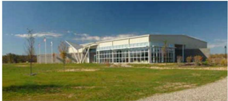
The Fernald Preserve Visitors Center (Source: US DOE)
