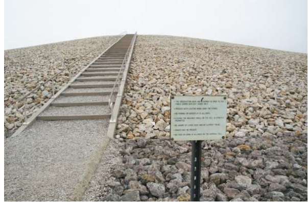
Stairway to an observation platform on 75-foot-tall permanent disposal cell
