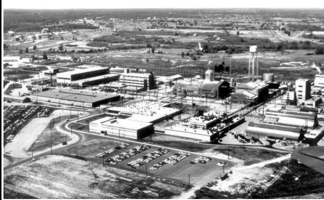
Weldon Spring Chemical Plant During Operations
