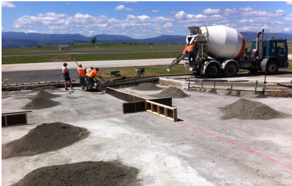
Construction of New Apron
