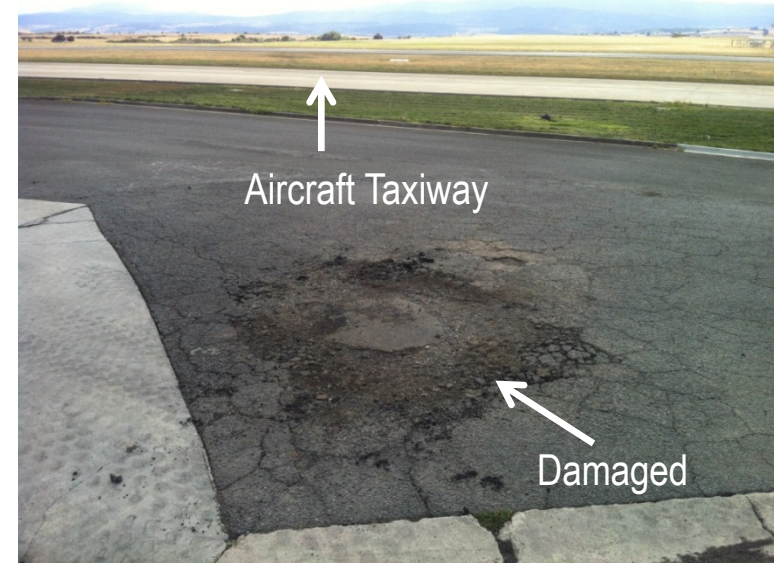
Damaged Asphalt
