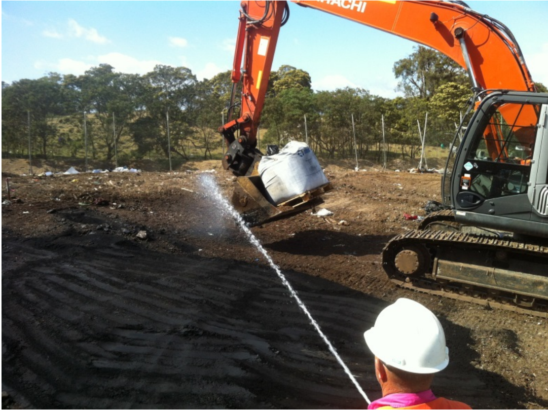
Laying the Amendment Capping Layer
