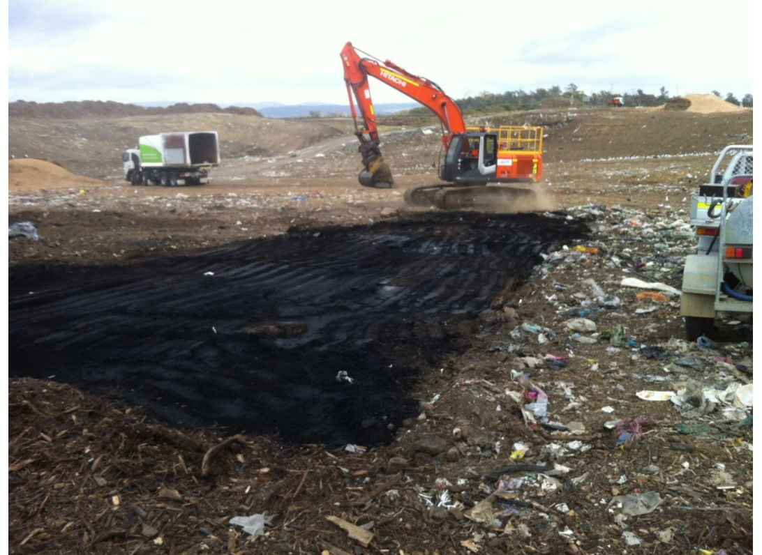
Finished Lined Burial Cell
