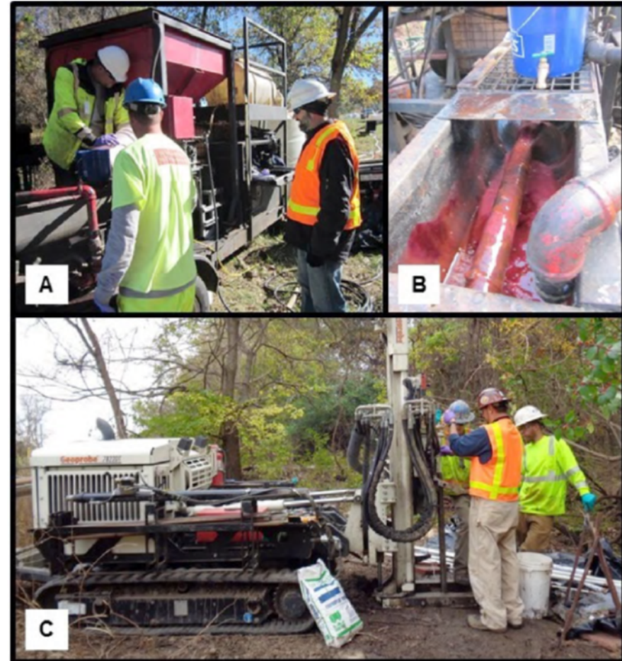
(A) Customized sand lens injection equipment. (B) Guar-sand injection solution with rhodamine dye. (C) DPT installation of sand lens.
