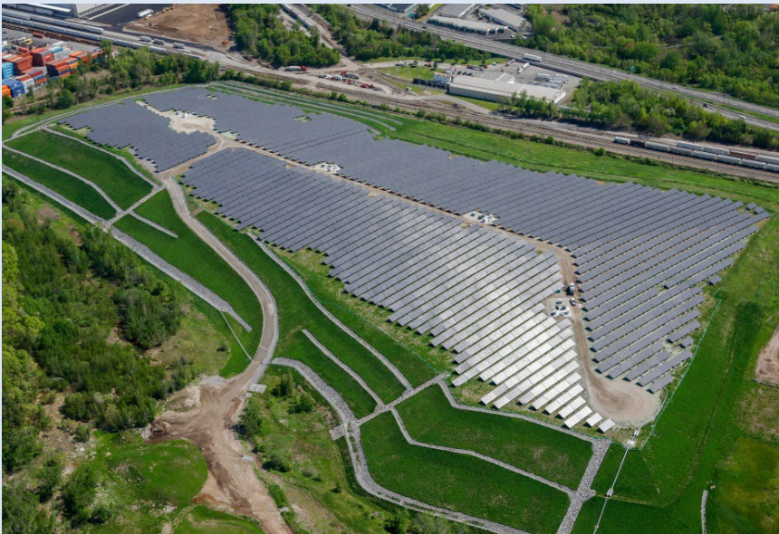
Greenwood Street Solar Farm in Worcester
