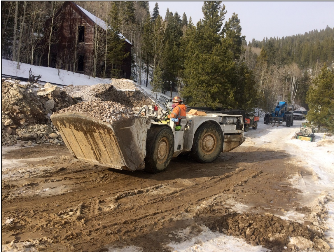
Mucker loading limestone into tunnel
