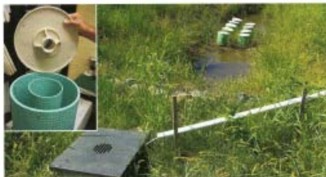
Right, top: Cartridge used with slag on Maryland's eastern shore sites. Right, middle: Box filters containing slag at a poultry farm. Right, bottom: A confined bed slag filter under construction on a golf course in Stillwater, OK.
