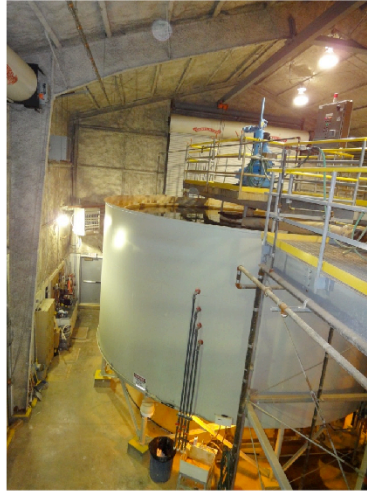
Clarifier in HDS system
