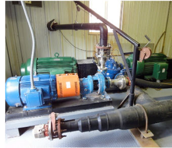
Strawberry Pump Station 68
