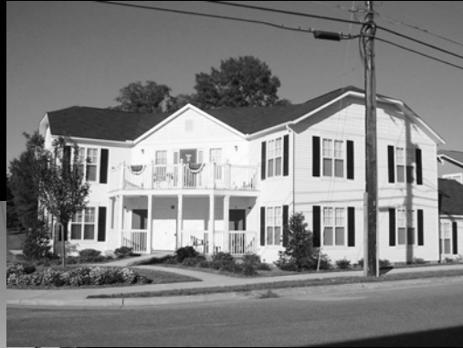
The Bungalows: 6-unit corner building
