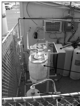
Effluent stream Heater control Propane Catalytic converters SVE pump
