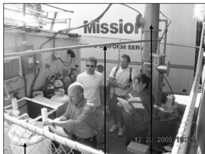
Catalytic converters Effluent stream Scrubber
