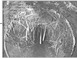
Deteriorated pipe
