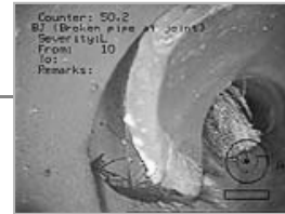
Broken and displaced pipe
