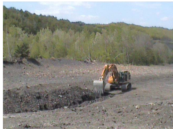
A backhoe is used to prepare the deep rows.
