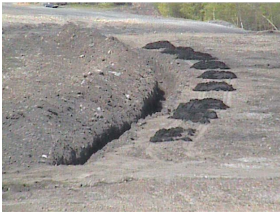
Surface mine with deep rows prepared for biosolids placement. May, 2005
