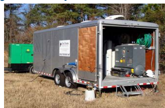
EnChem Engineering PFAS Treatment
