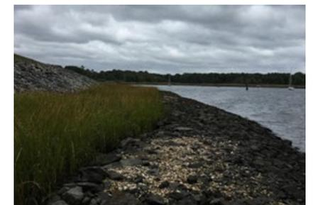
*Revetment, constructed wetland and breakwater structure*
